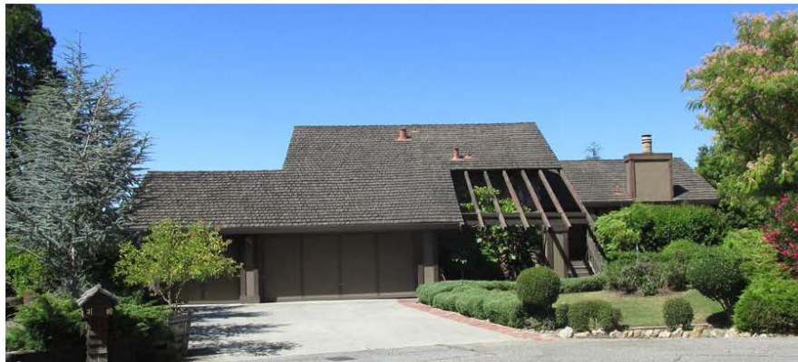
Photo 5. Combustible Wood Roof.
